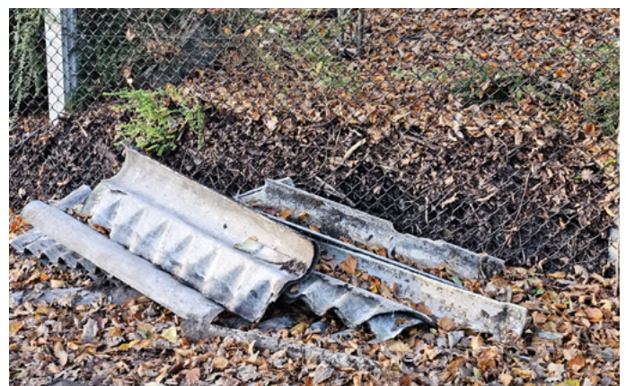
Fig 2. Asbestos containing corrugated cement sheet, commonly found on garage roofs)
