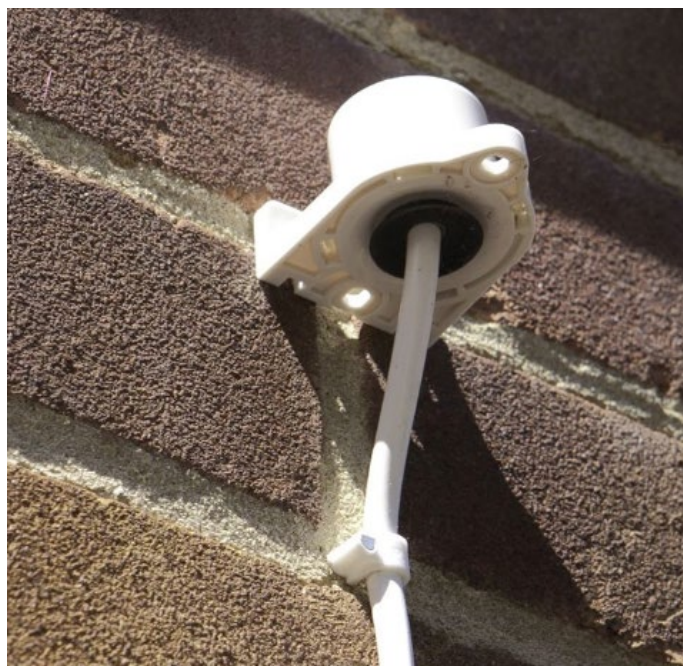
Figure 5 - Weather compensation outside sensor
