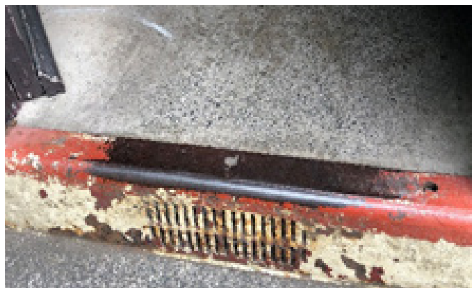
Figure 6 - kerb to support the original floor joists (since concreted as part of the modernisation works)
