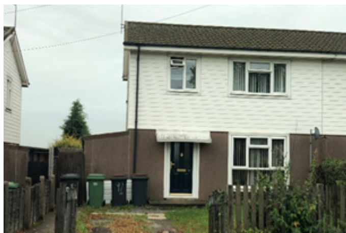
Figure 7 - Example of BISF house
