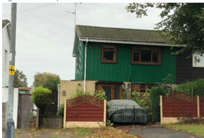
Figure 8 - Example of BISF house
