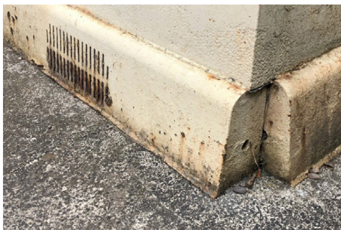
Figure 5 - splayed concrete ground beam
