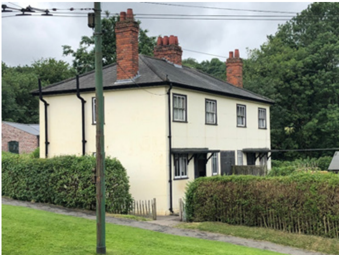
Figure 1 – semi-detached cast iron houses in Dudley
