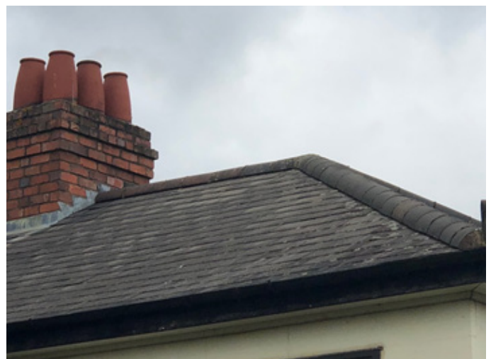
Figure 2 – Welsh slate roof
