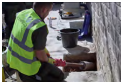
Figure 1 - radon sump installation
