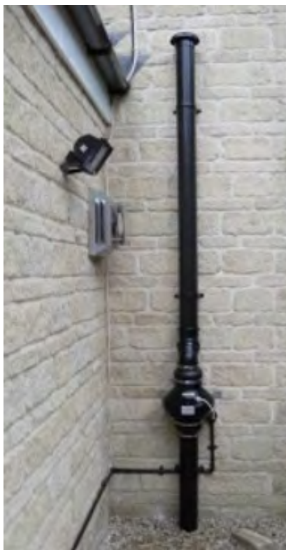
Figure 2 - example of exhaust pipe
