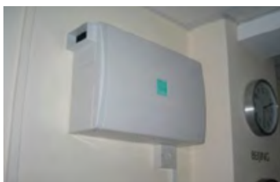
Figure 3 - example of a positive pressure system
