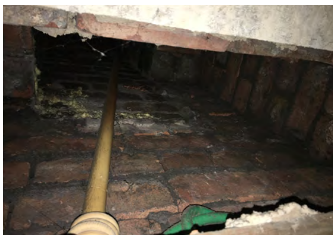
Figure 2 – bottom of chimney stack opened.
