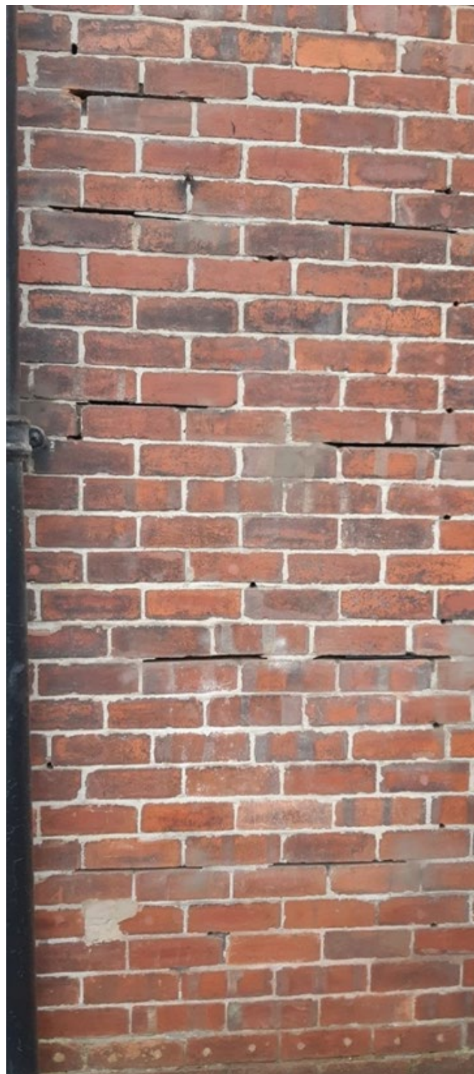
Figure 8: Horizontal chases in outer leaf wall
