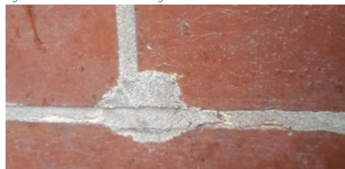
Figure 13: Drill hole evidence through mortar
