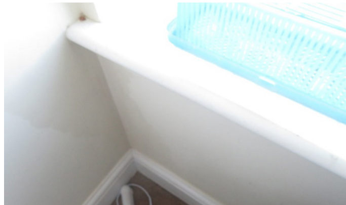
Figure 8: Water marks visible
