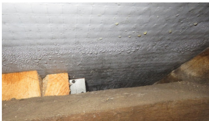
Figure 10: Condensation to rafter felt
