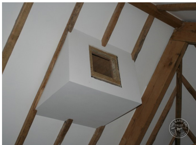
Figure 7: Internal access of the barn owl nesting box. Copyright: The Barn Owl Trust
