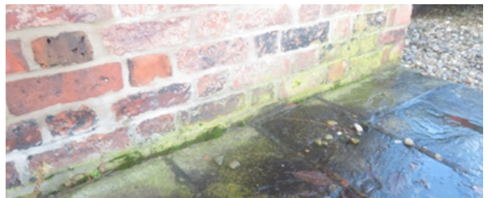
Figure 2: Biological growth externally
