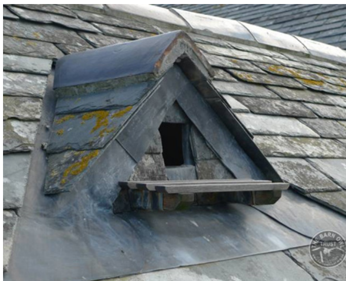
Figure 6: External view of barn owl nesting box built into roof structure. Copyright: The Barn Owl Trust https://www.barnowltrust.org.uk/
