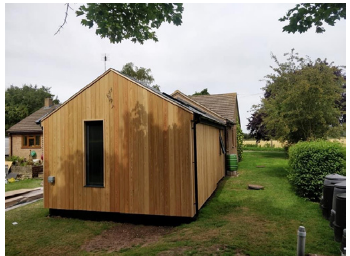
Figure 2: Example of structure using ground screws
