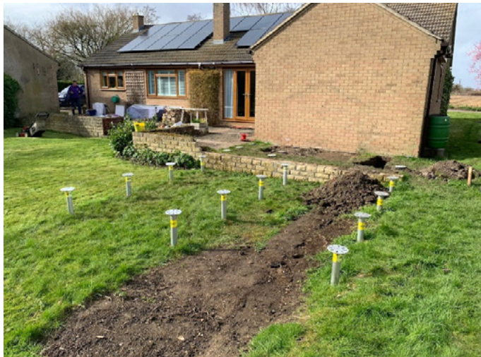
Figure 1: Ground screws placed in position
