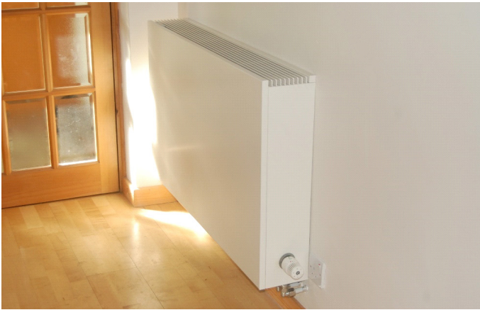
Figure 4: Example of a radiator used with a heat pump. Source: Jaga UK
