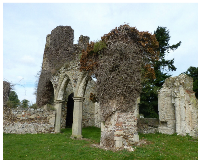
Figure 1: Appleton Church before restoration
